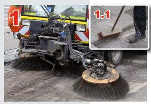
Prior to laying the BORNIT® Joint Tape, the substrate is freed from dust or loose particles (Image 1). A clean and solid substrate facilitates assembly.
