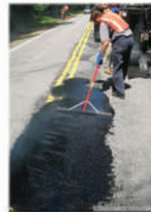
Repairs prior to surface treatment
