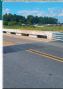
Bridge deck approach
