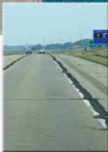
Longitudinal cracks ( \geq 1.5" )
