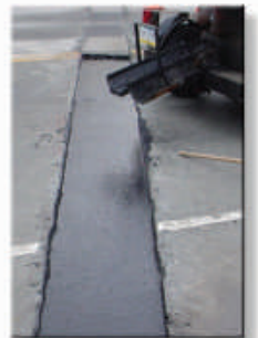
Leveling utility cuts
