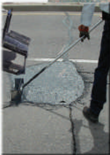
Patch deterioration & pothole repair
