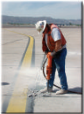
Clean Out Old Material
